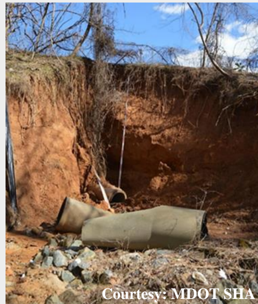
Figure 2. Examples of Severe Outfall Erosion in the Headwater Transition Zone
